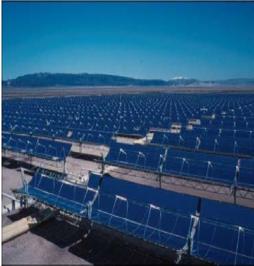
Parabolic trough collector field for the solar thermal power plant at Kramer Junction, California
